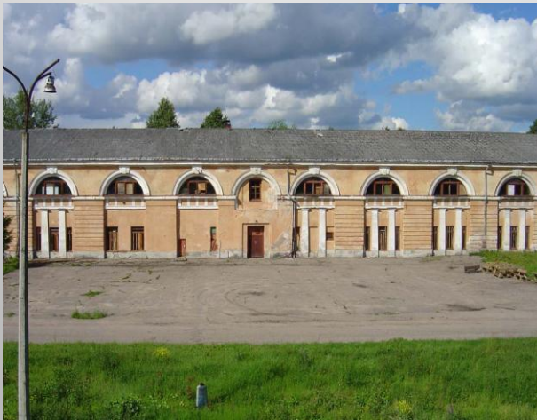
Military arsenal building
