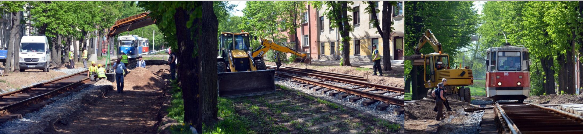
Reconstruction of rails and acquisition of tramcars
