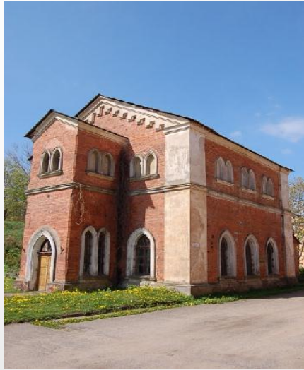
Old Water Tower
