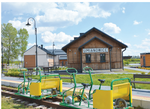
Nature Education Center in Umianowice, Railbike
